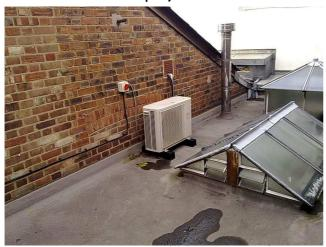
of these was the fitting of a covering layer of specially designed material to the flat roofed section, extending its life by an estimated 20 years. In addition a series of general repairs was carried out including glazing repairs, redecoration of woodwork, and repairs to flashings, slates, and mortar. This planned preventative work has put the roof in excellent order and means that no further major roof repairs are likely to be needed for some years.
